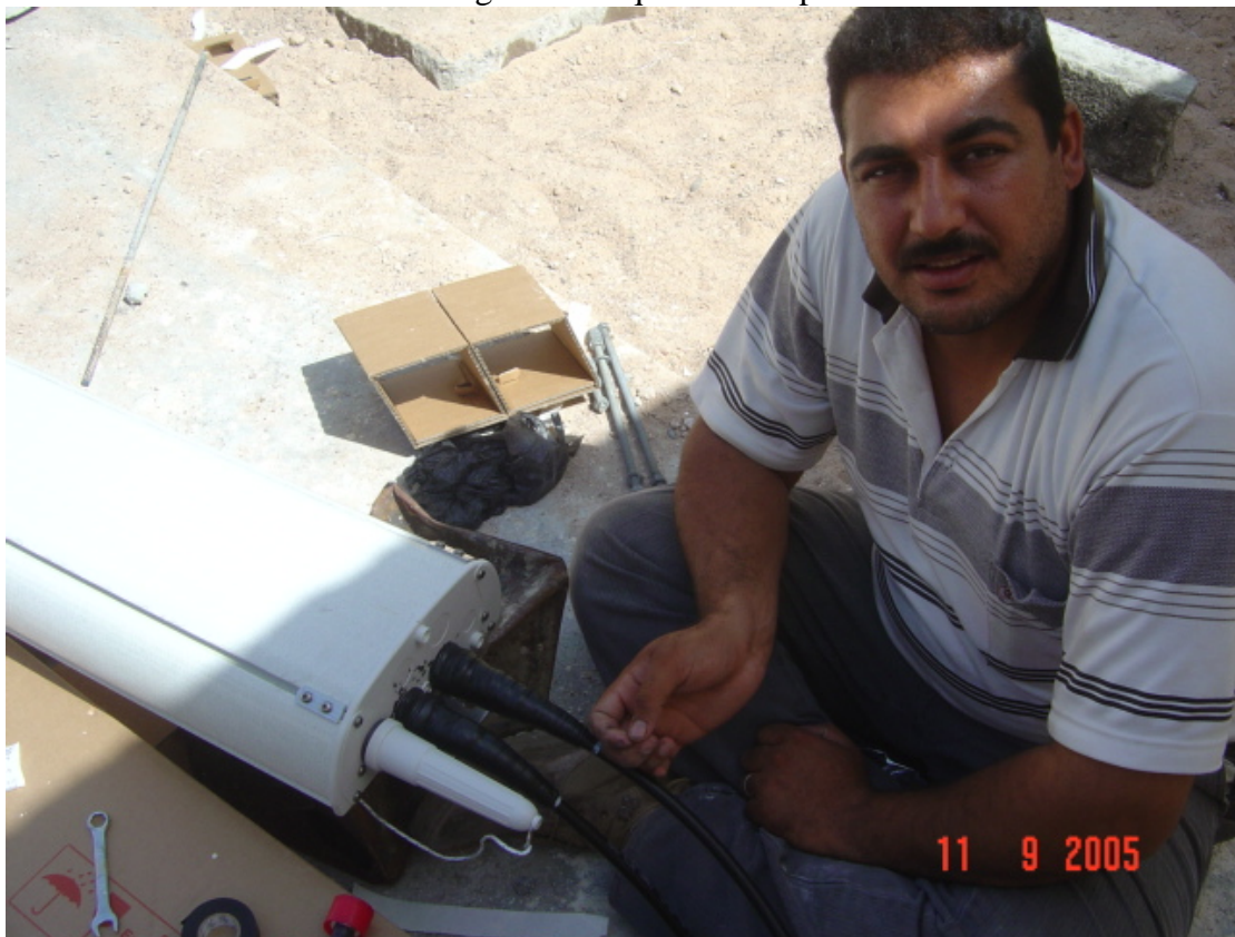
Through RF work
